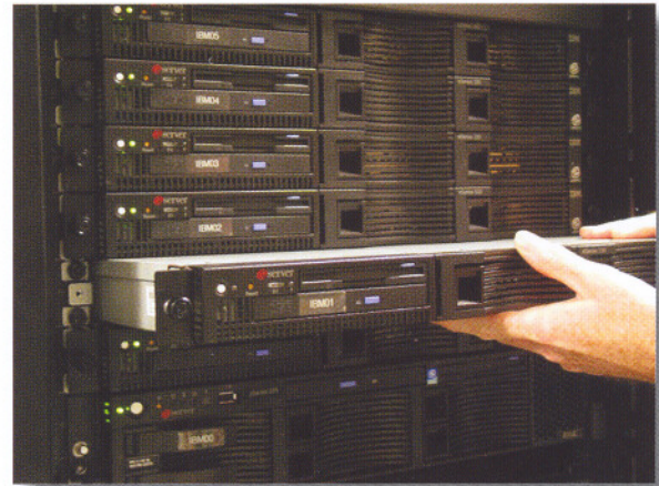
Replacing a defective member of a cluster.
